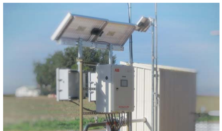
A high IO count Totalflow XSeries powered by solar charged batteries
