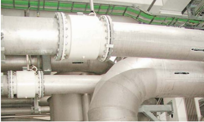
Metering pulp in a paper mill
