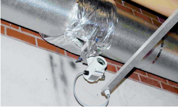
OriMaster M installed in a lagged steam pipeline
