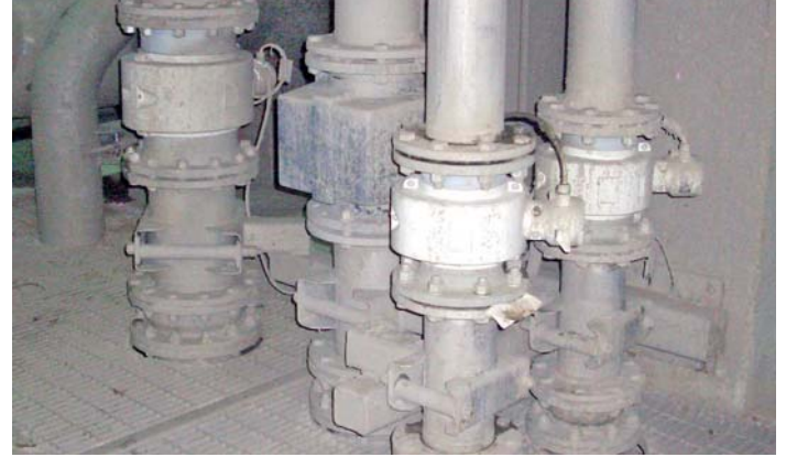
Metering reject in a paper mill
