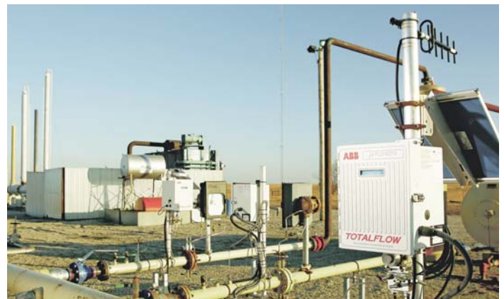
Totalflow XSeries RTU in a natural gas multi-well PAD application
