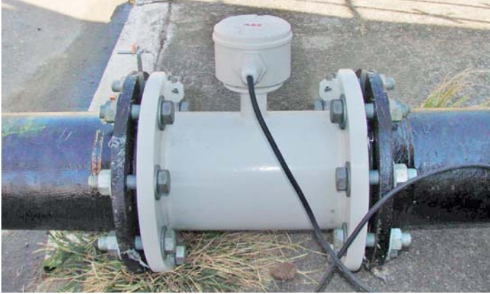
AquaMaster reduced bore flow sensor installed in potable water network
