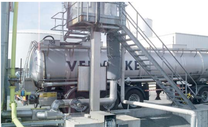
The CoriolisMaster sensor in a custody transfer truck filling application
