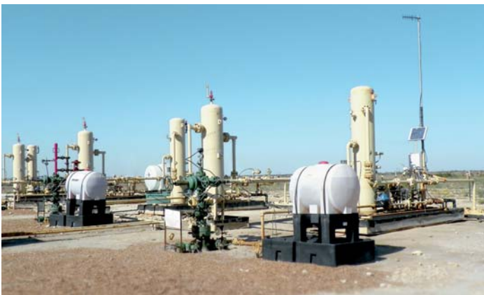
Real time automation of chemical injection
