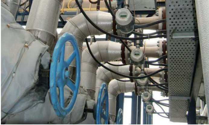
Space saving swirl meters in steam application
