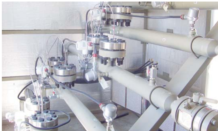
Wedge flowmeter in wellhead natural gas application
