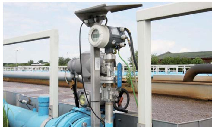
Sensyflow FMT500-IG at a water treatment plant
