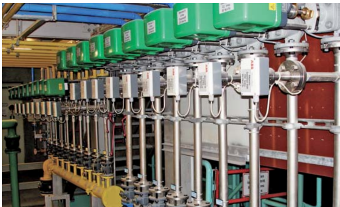
Sensyflow FMT400-VTS for precise burner control
