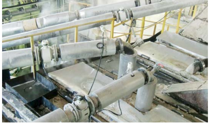
Hot fluid measurement with ProcessMaster in a chemical plant
